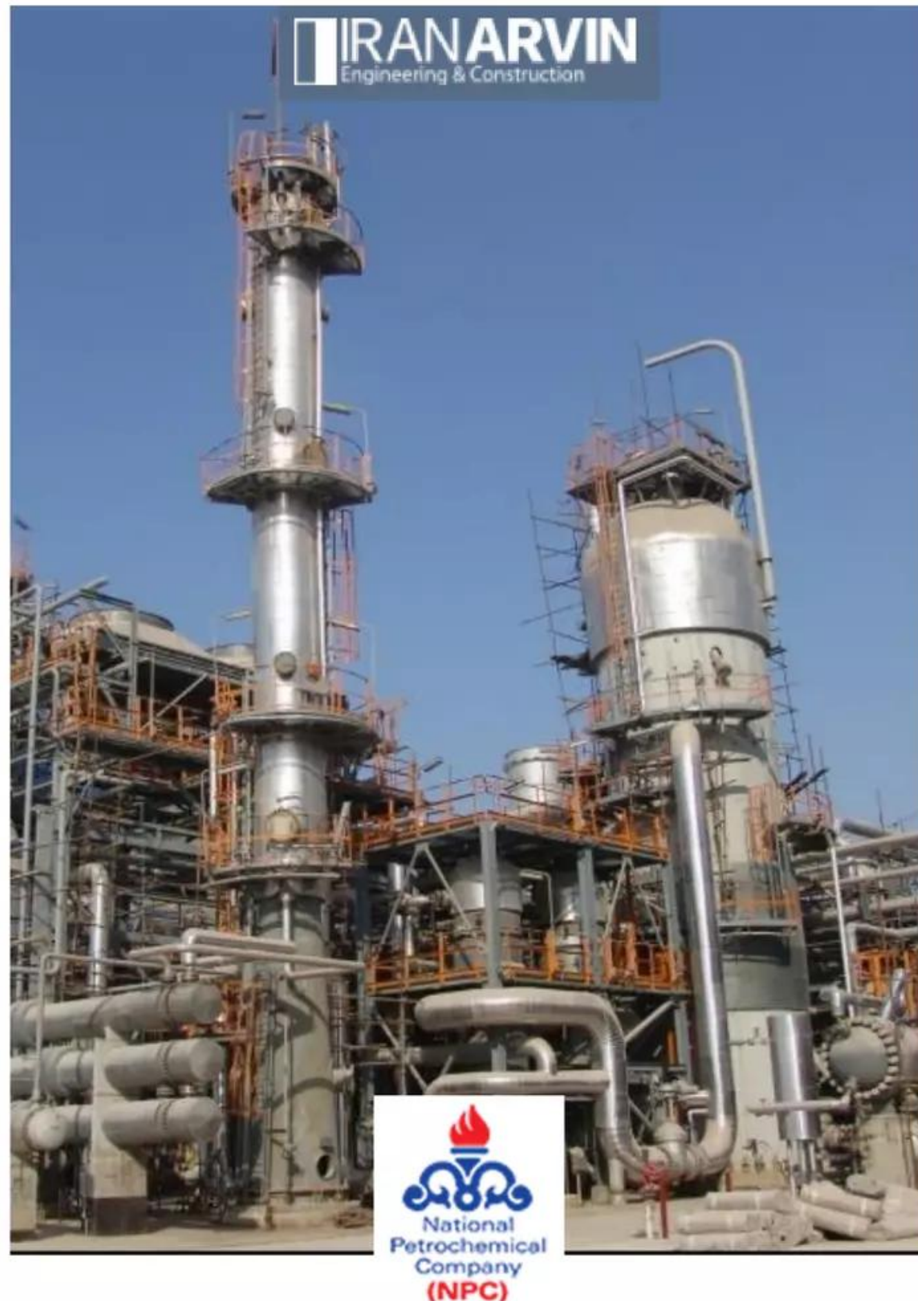
Reactor on left \sim 100 feet tall
